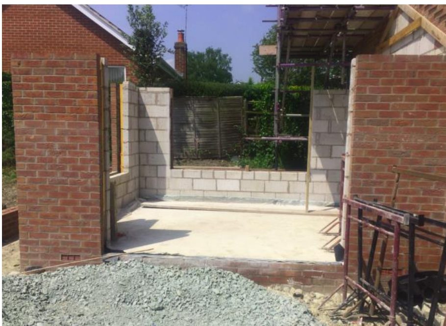
Fig 3 - Conservatory window opening
